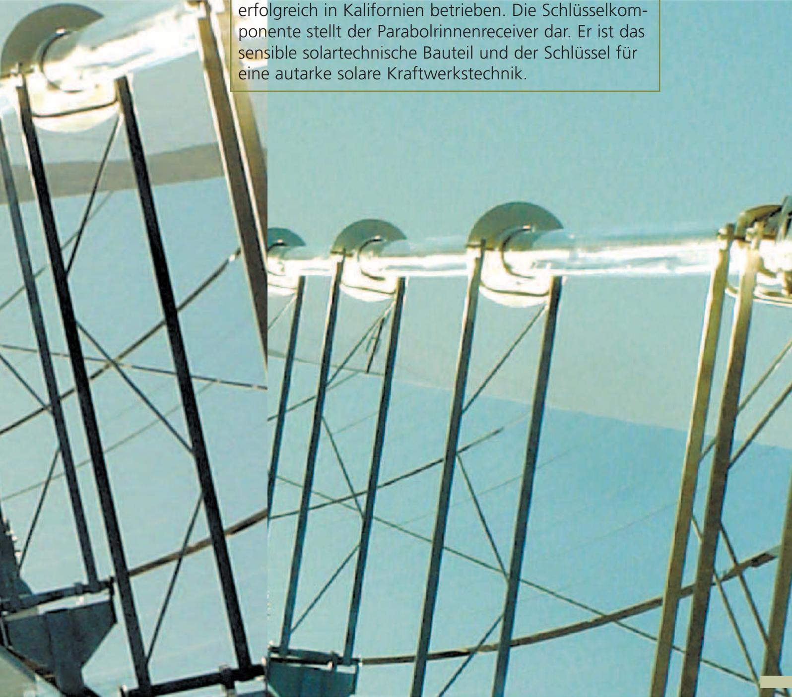
A close-up photograph of a parabolic trough receiver, a key component of solar thermal power plants. The receiver is a long, cylindrical metal tube with a highly reflective, polished surface. It is supported by a complex metal truss structure. The background shows a clear blue sky and the structural elements of the tower. The receiver is positioned to capture and focus sunlight onto a central receiver tube.
