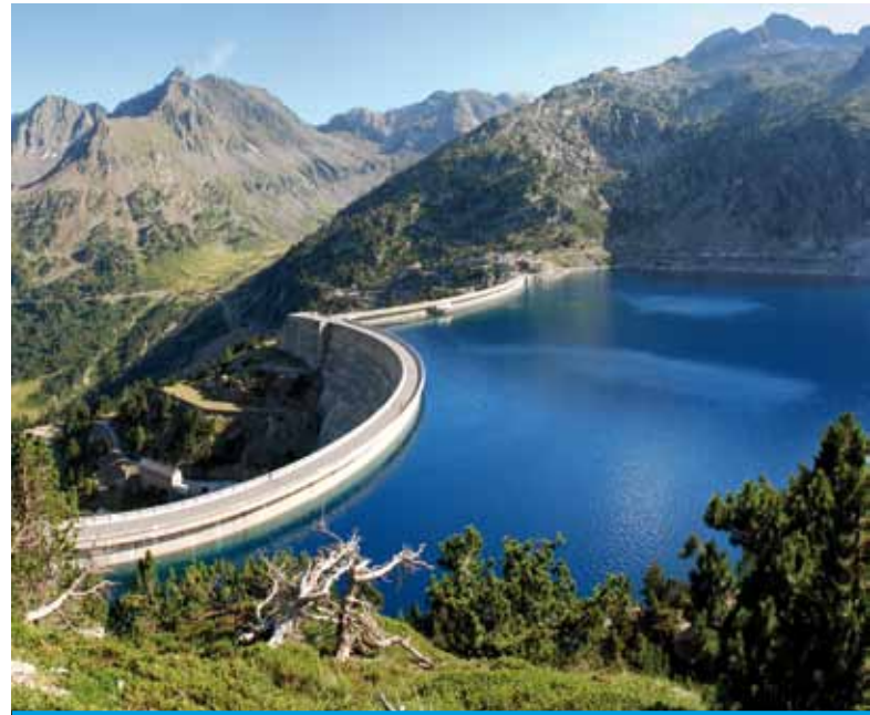
Water reservoir Lake Cap-de-Long (France)
