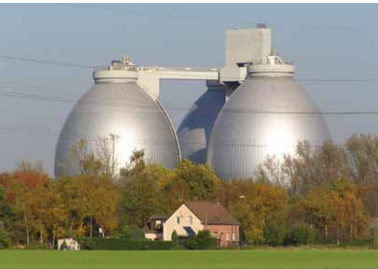
Anaerobic digestion tanks, wastewater treatment plant "Emschermündung" (Germany)
