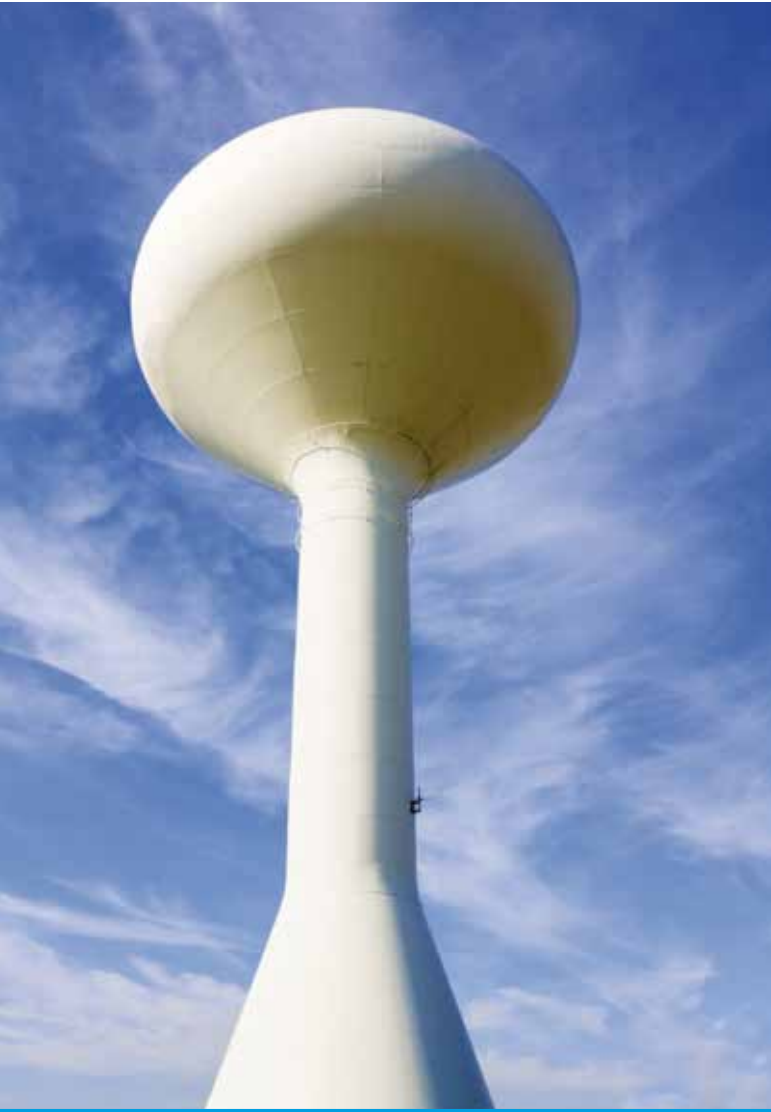
Water tower stores clean drinking water
